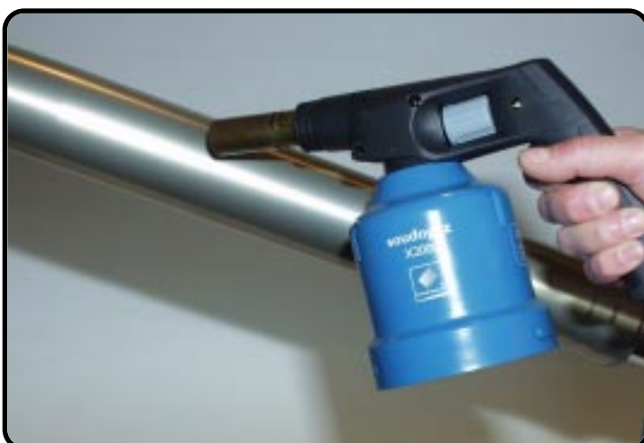
Heat the outer-tube at this level..
